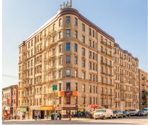
St. Nicholas Manor | Manhattan, NY | 112 units | Section 8
